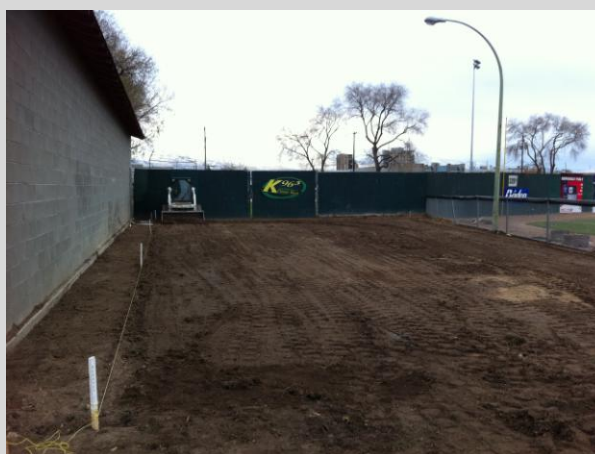
Netex Center for Hitting Site Preparation November 26 th , 2011- Phase 1
